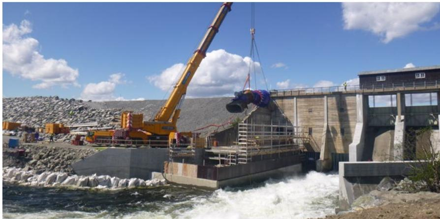
With its Kaplan S bulb turbine, Kössler was able to offer the optimum solution for the strongly fluctuating head and received the order together with Voith Hydro in Oslo. The plant was designed in such a way that its operation is maintai-
